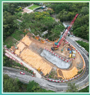
土地平整 Site Formation Works
