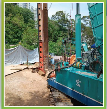
挖掘及側向支撐工程 Excavation and Lateral Support Works
